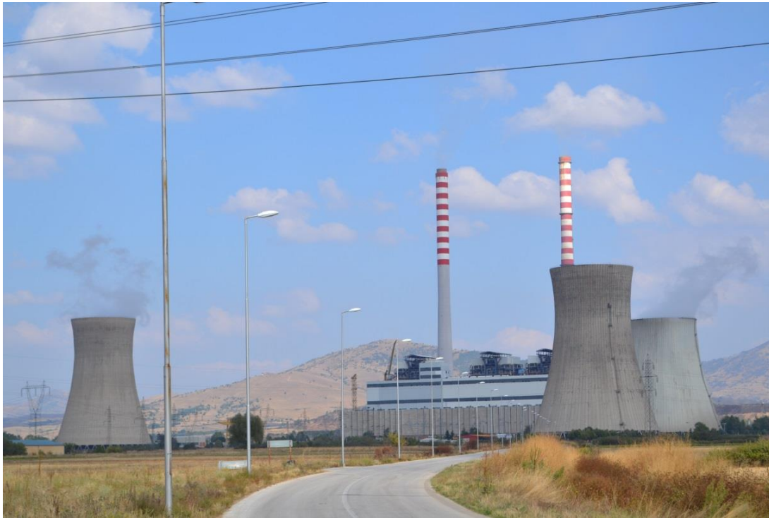
Figure 21. Coal powered thermal heating power plant REK Bitola (Photo: MEPP, 2016).
